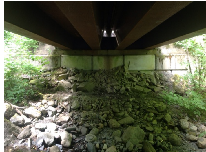
Left Bank Abutment when facing downstream
