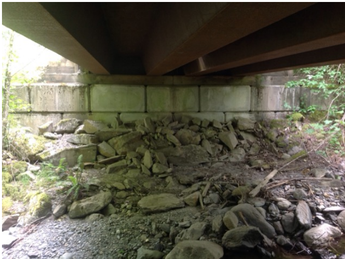
Right Bank Abutment when facing downstream
